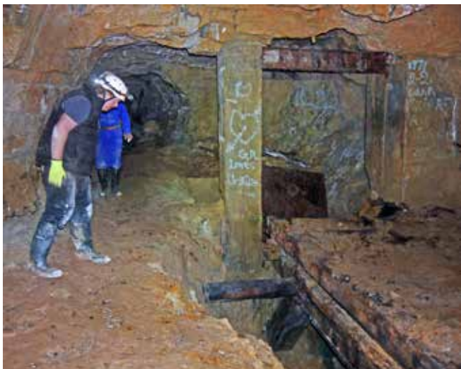
Contact shaft; the shaft is flooded below the lower adit level. Photo Ken Geddes
